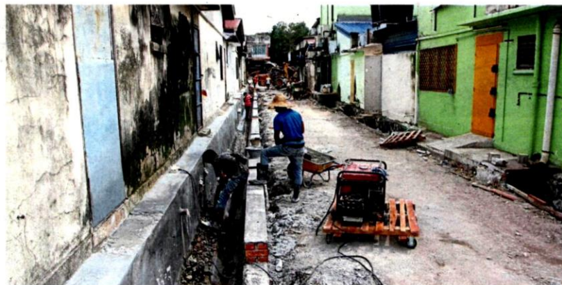
Some of the new drains are nearly completed. — Photos: LOW BOON TAT/The Star
