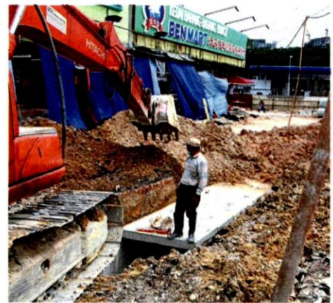
The upgrading work involves a lot of digging to widen and deepen the drains.
